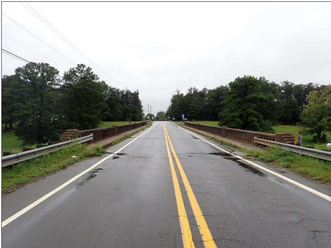
south approach looking north
