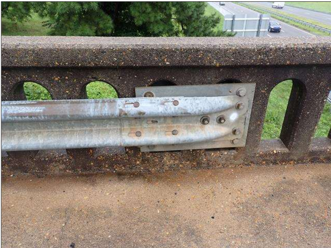
northeast guardrail attachment
