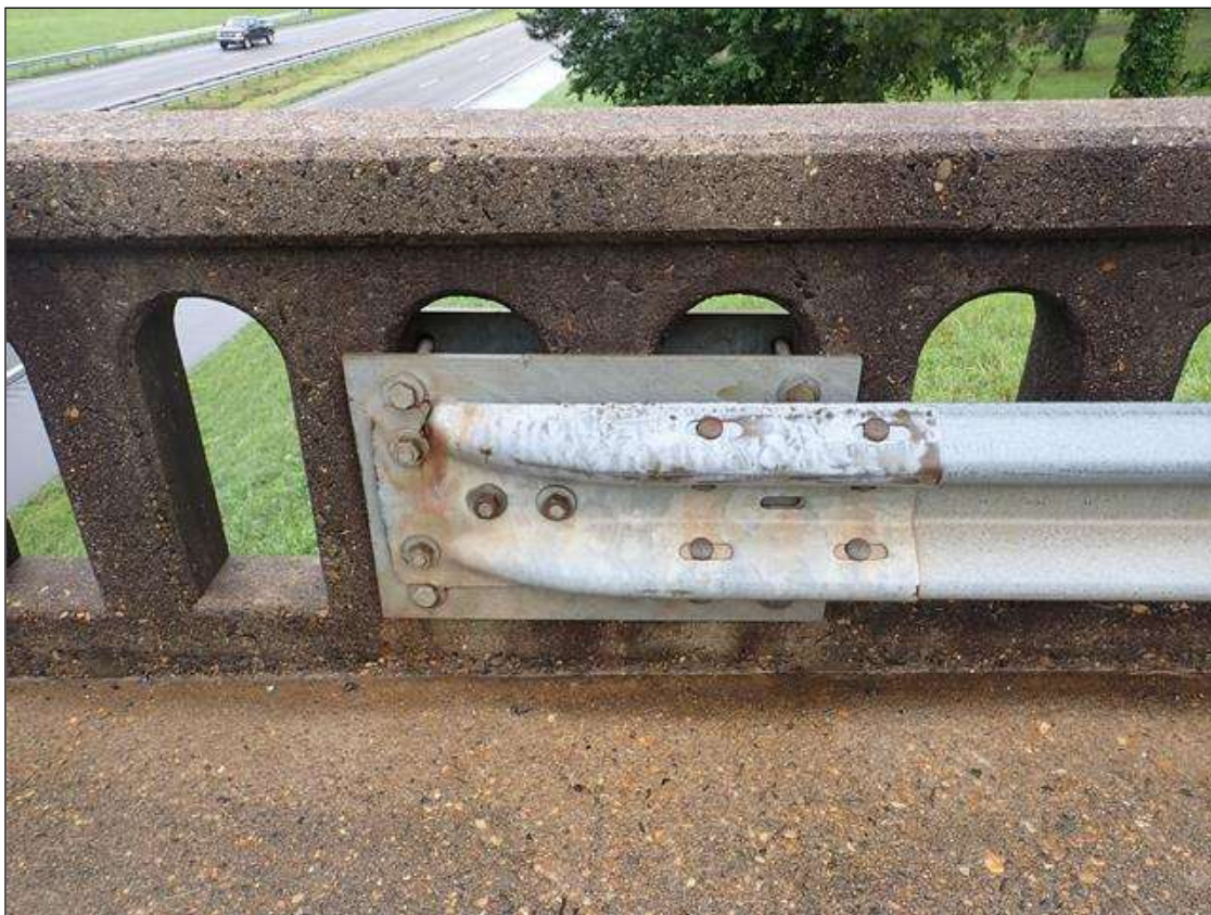
northwest guardrail attachment
