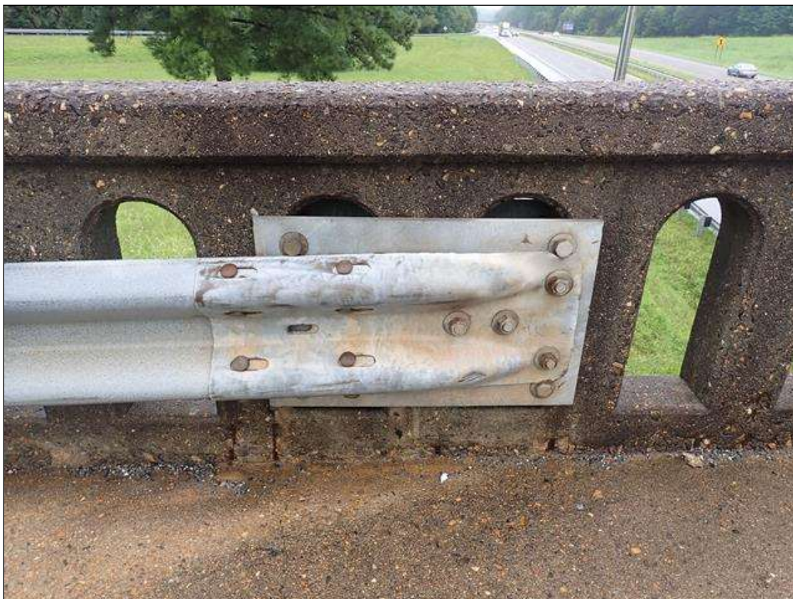
southwest guardrail attachment
