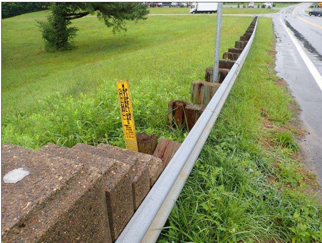
southeast guardrail transition
