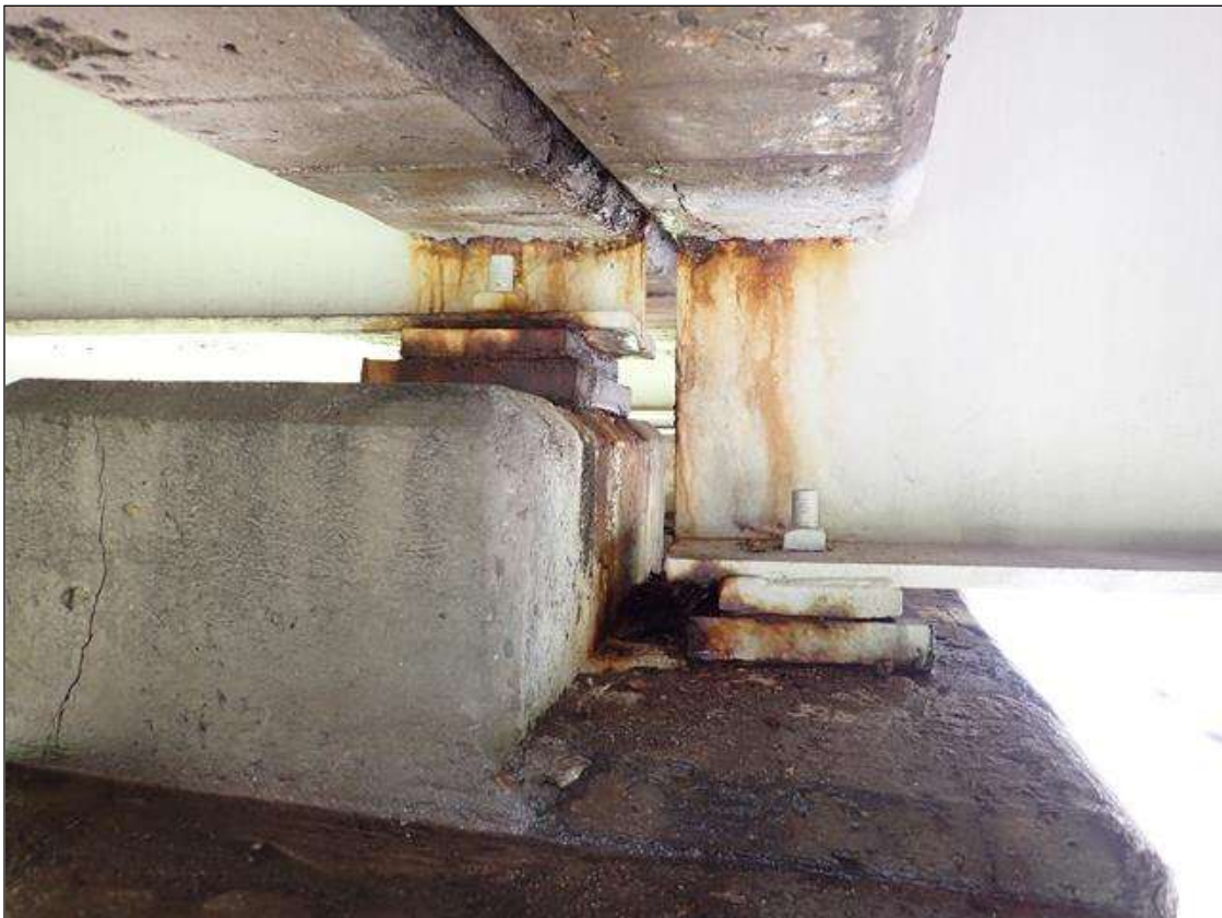
beams over bent 1 and interior bearing assembly (interior beams)
