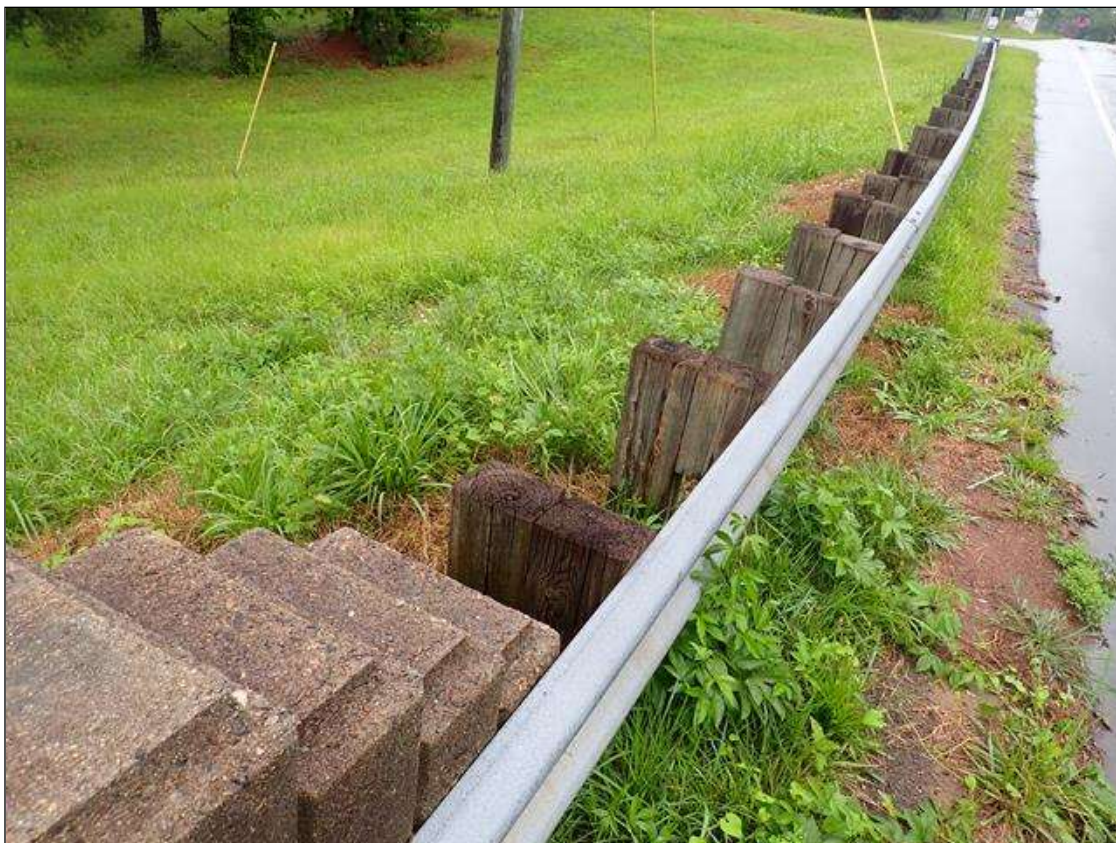
northwest guardrail transition
