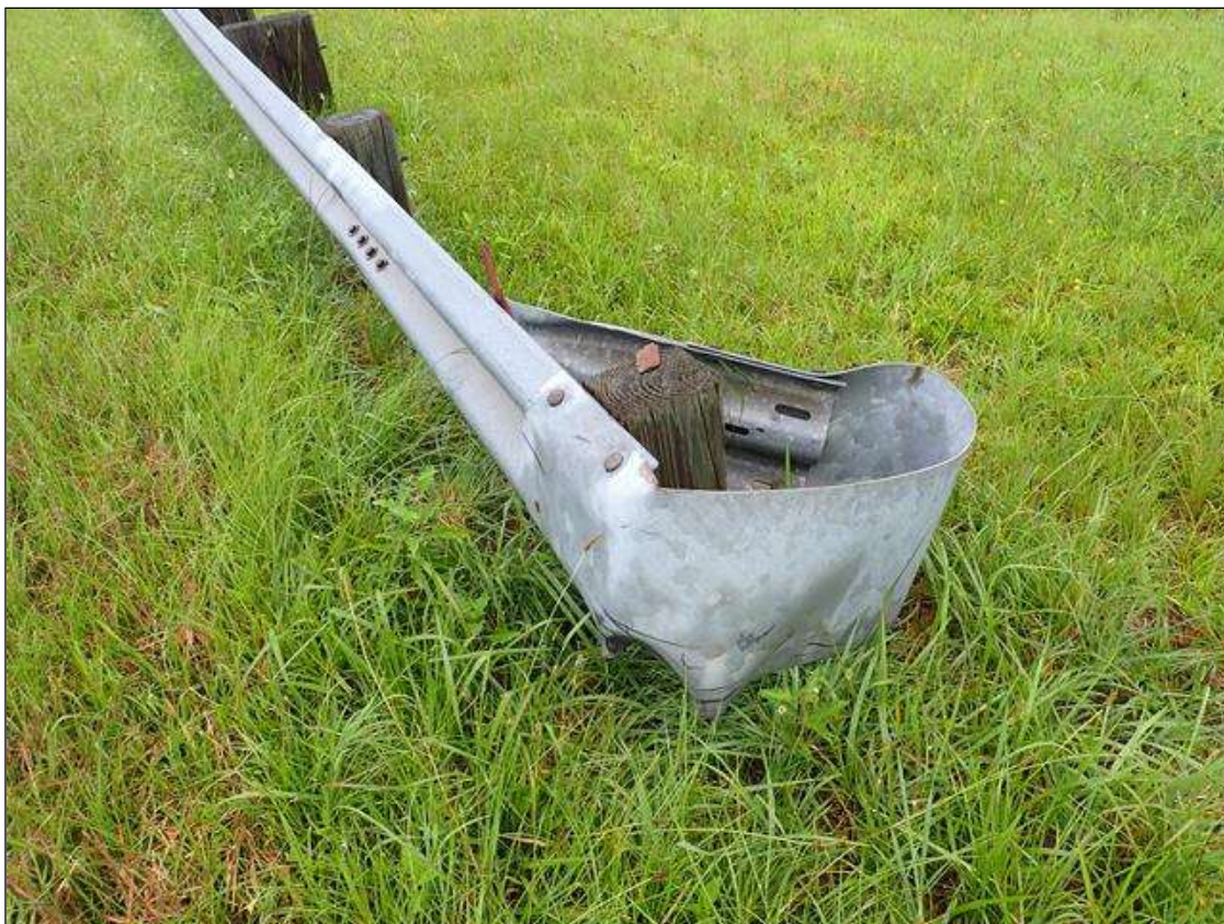
southeast guardrail termination
