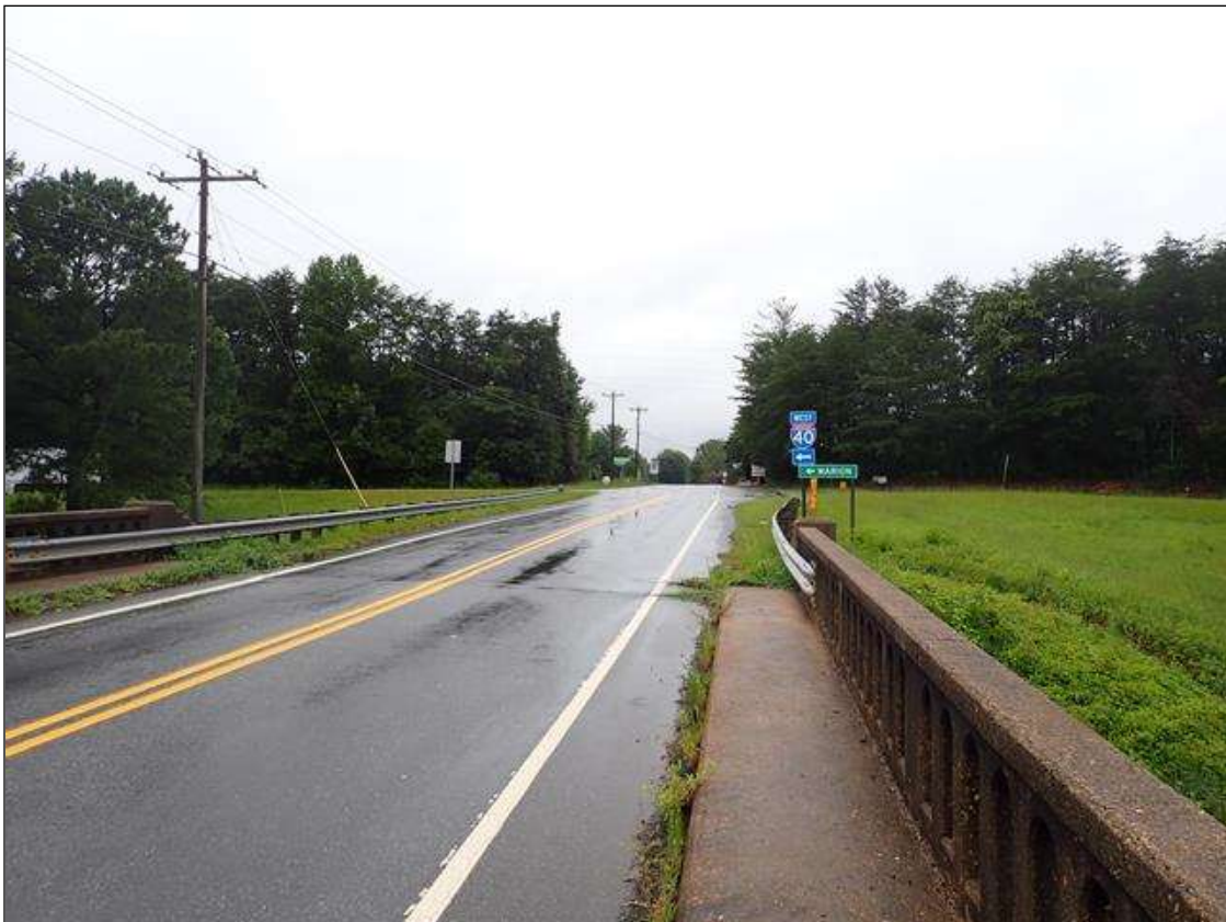
north approach looking north
