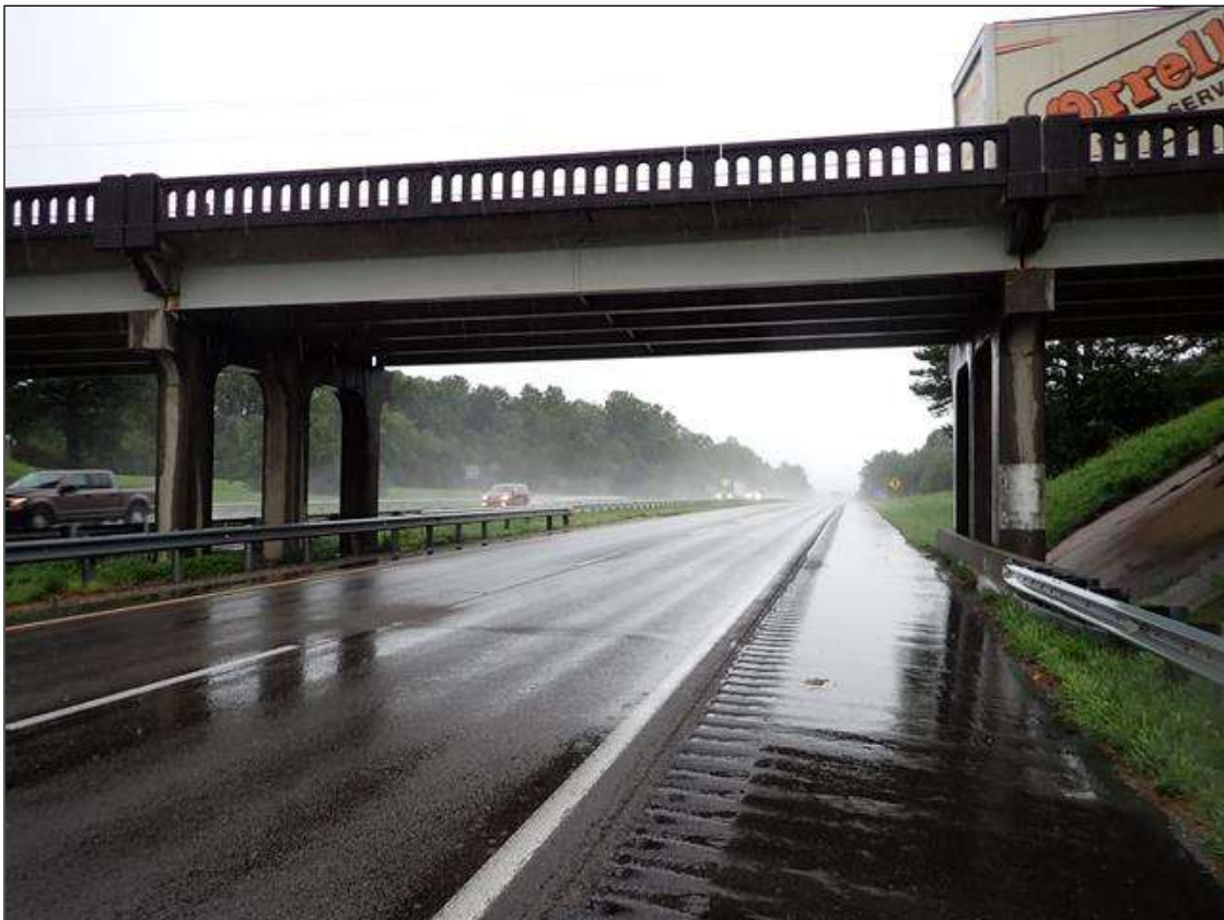
roadway under span 3, looking west
