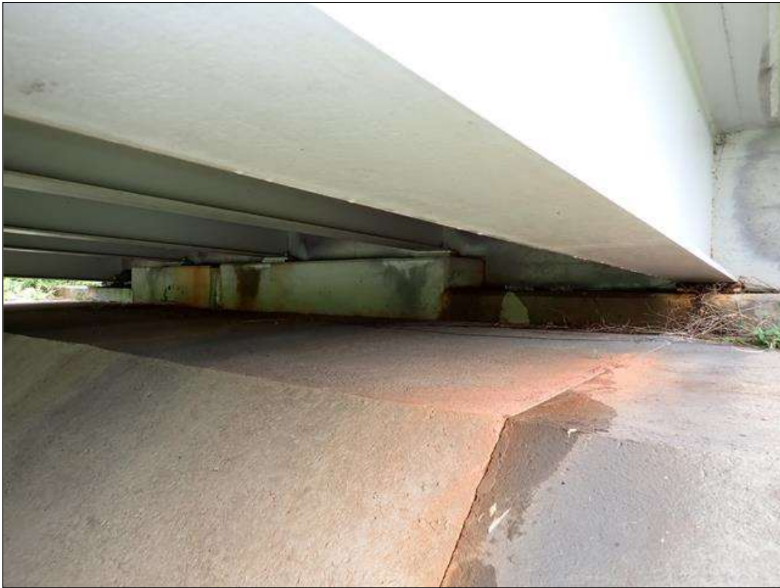
end bent 1 and slope protection
