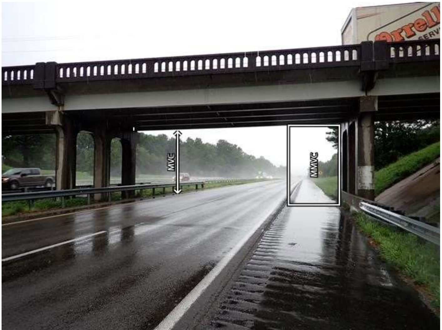
roadway under span 3, looking west
