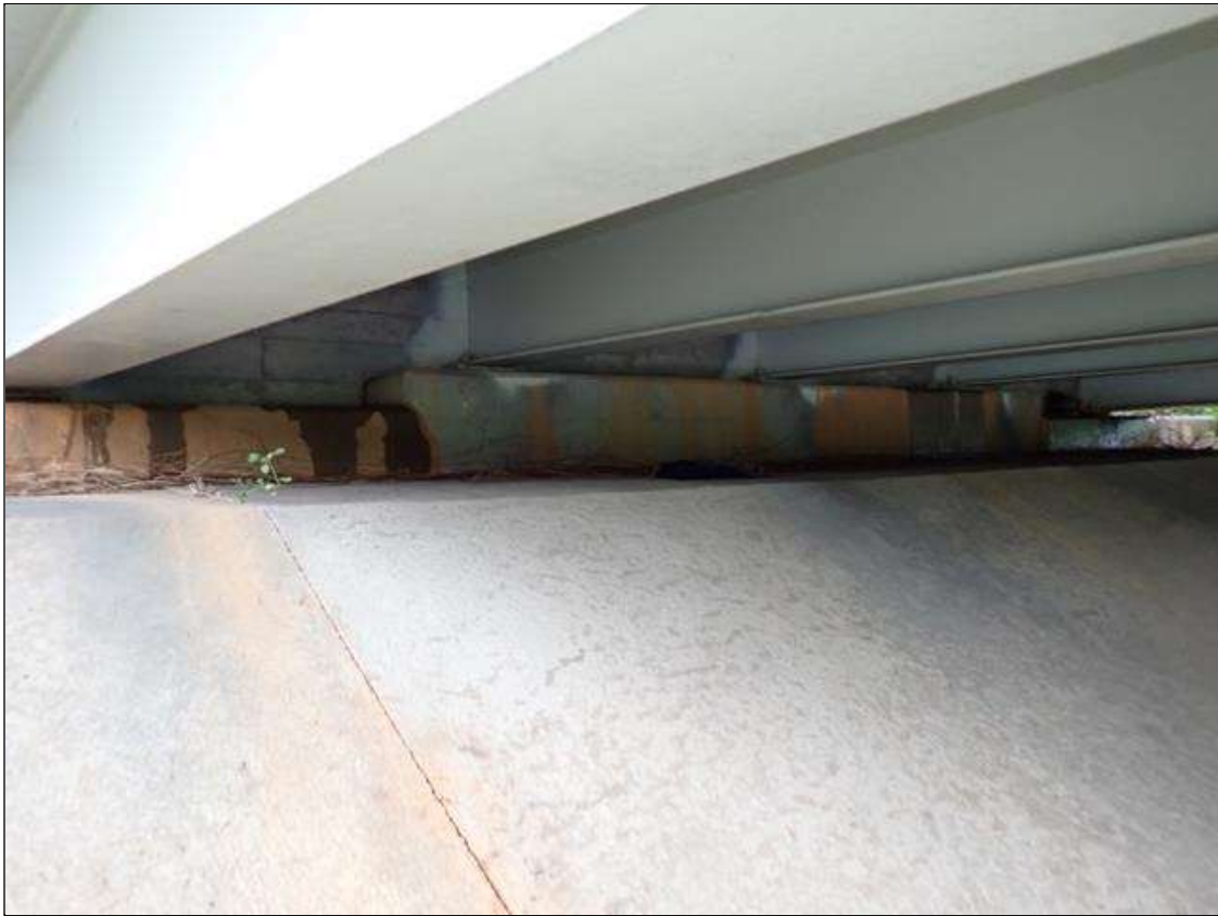
end bent 2 and slope protection
