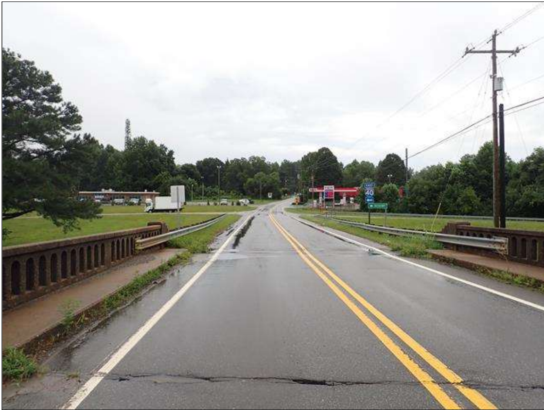
south approach looking south
