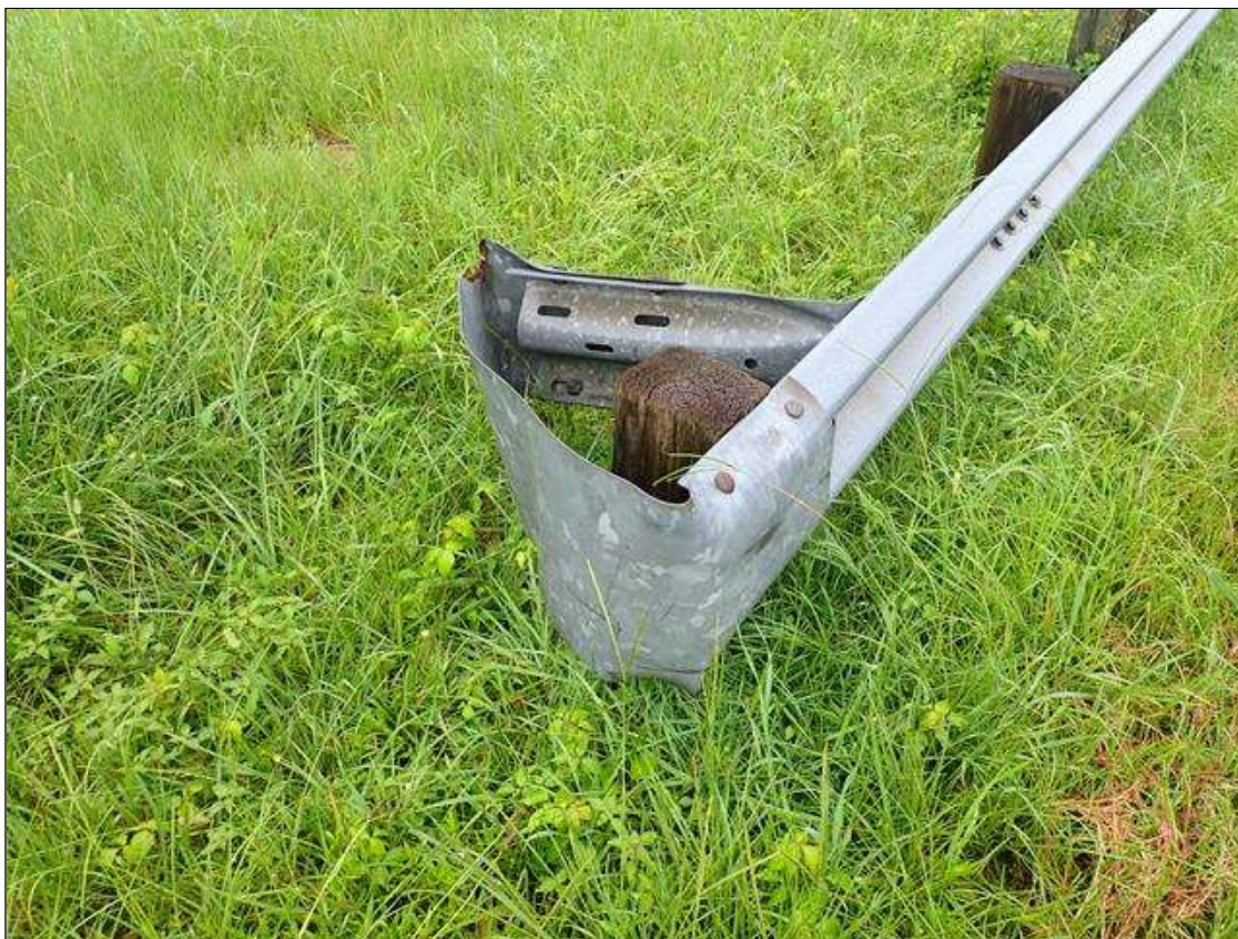
northeast guardrail termination
