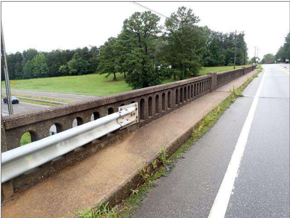
left bridge rail
