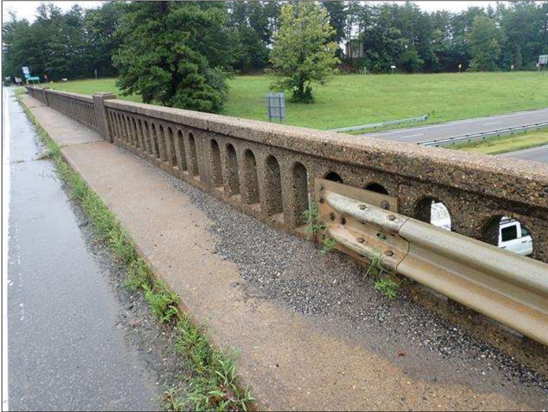
right bridge rail
