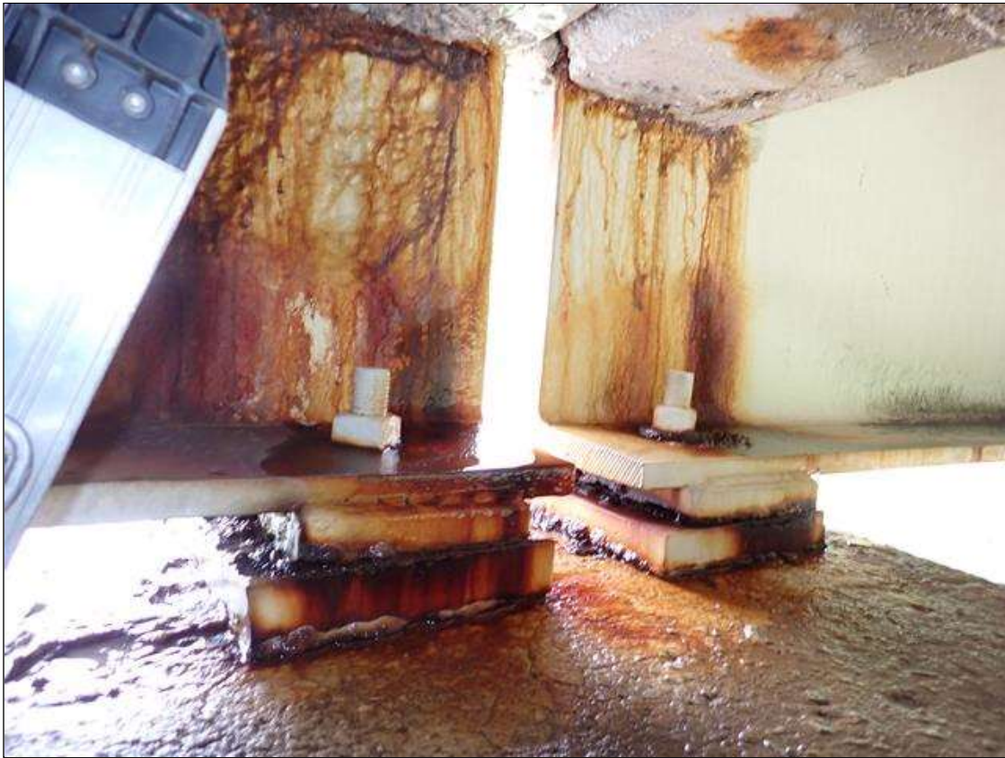
beams over bent 1 and interior bearing assembly (exterior beams)
