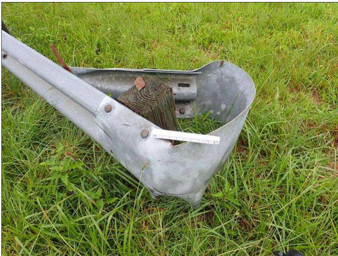
(PAR) southeast guardrail termination, impact damage
