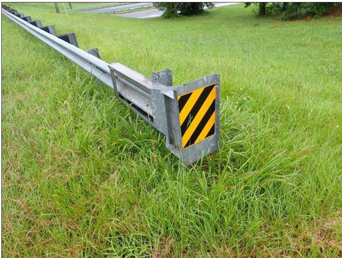
northwest guardrail termination
