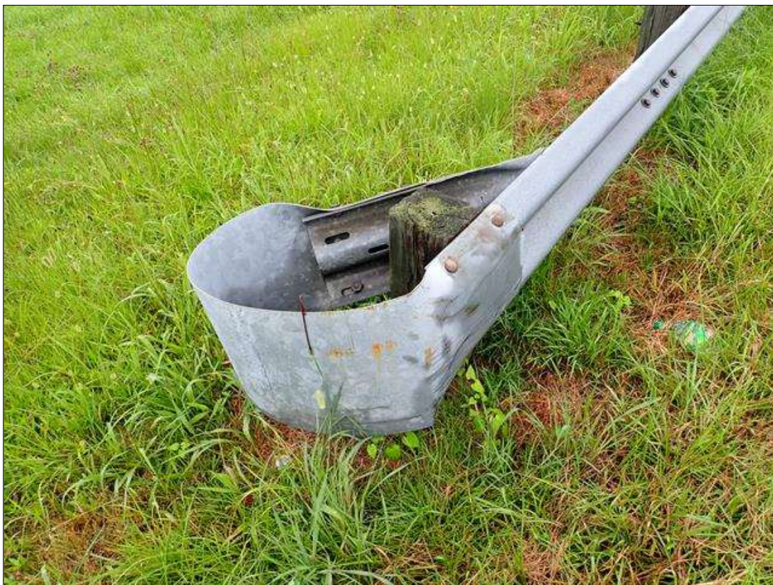
southwest guardrail termination
