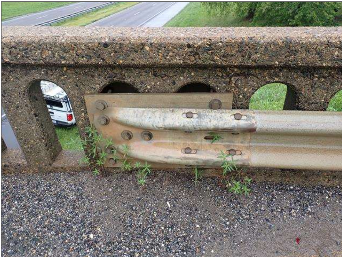
southeast guardrail attachment
