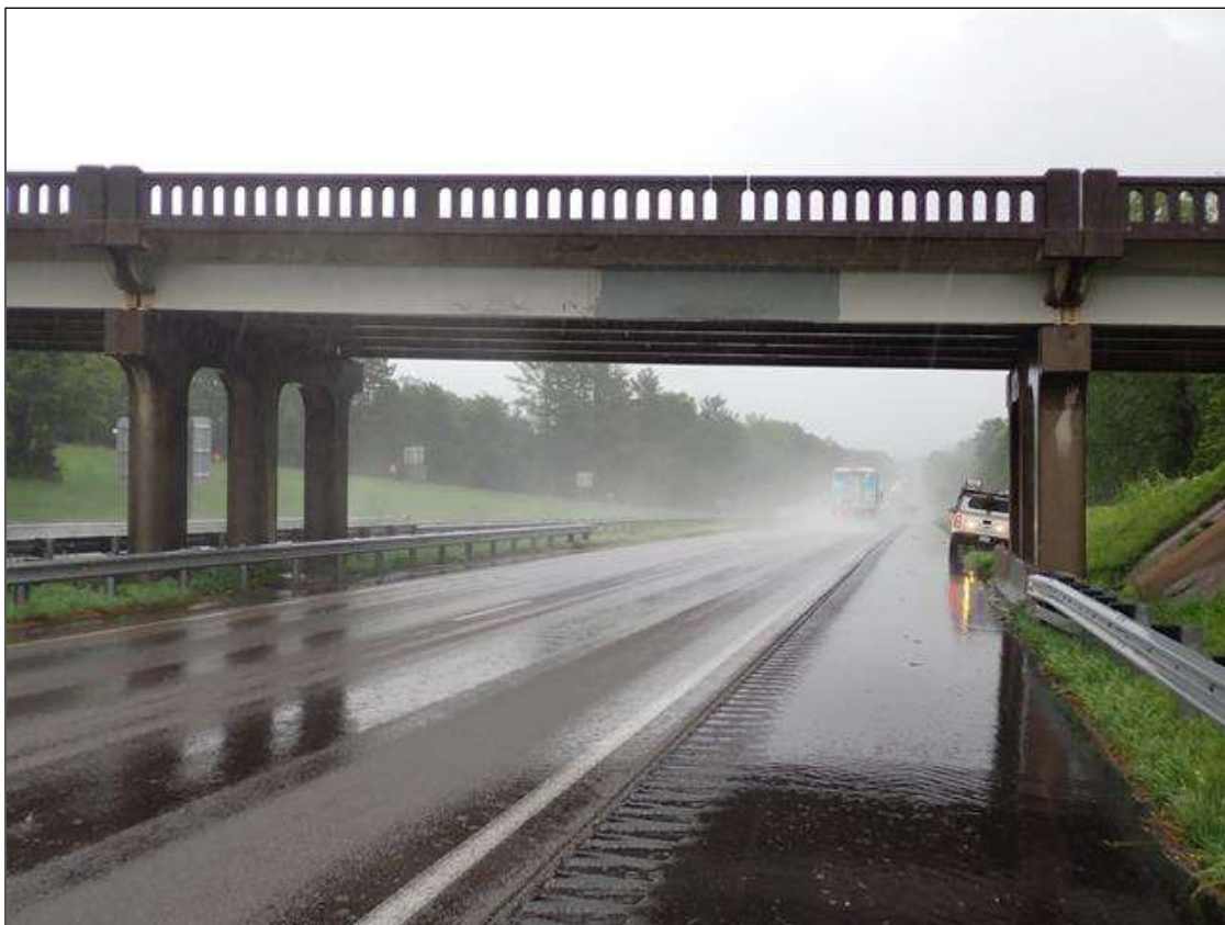
roadway under span 2, looking east
