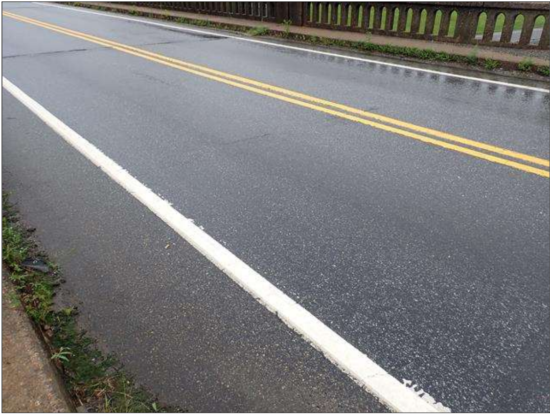
asphalt wearing surface
