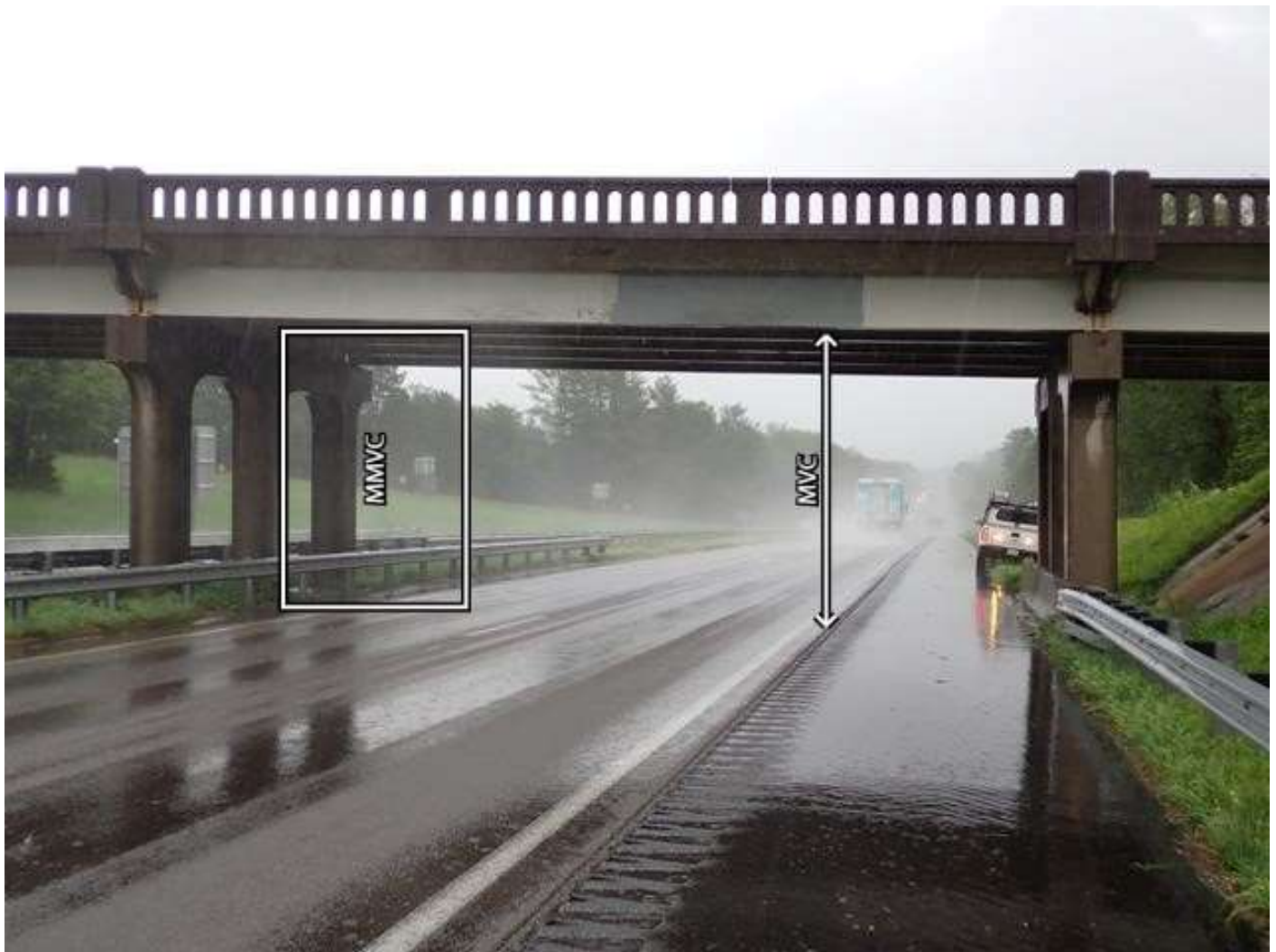
roadway under span 2, looking east
